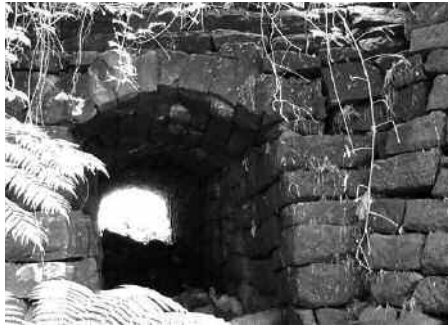
Eastern arch of The Bulwark bridge. Photo: Jon Kirkwood
