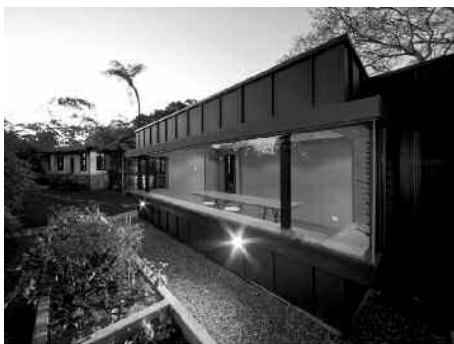
The studio extension to the Hugh Buhrich wing of the Cheong House at 14 The Parapet. Photo courtesy Willoughby City Council.
