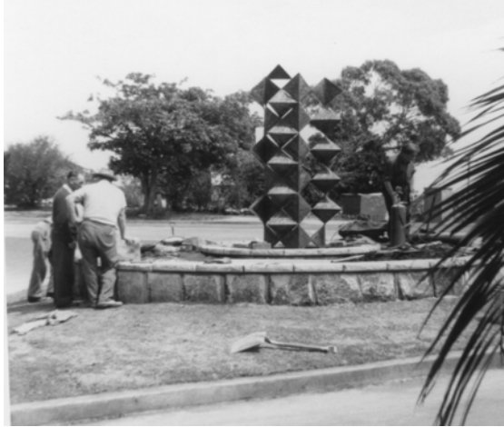
Construction of the Griffin Memorial Fountain in 1965. Note the crystalline shapes in freeform nodules of copper. Photo: Harry Fox
