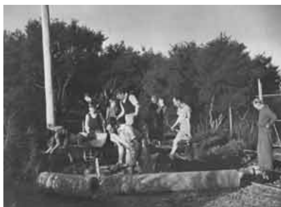
Castlecrag residents undertaking preparation work for their new Community Centre
