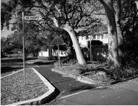
The restored traffic island (right) and the new garden area (left). Council has offered to take the smooth top off the new sandstone to achieve a natural finish in keeping with other sandstone elements in the Conservation Area. Bob McKillop photo.
