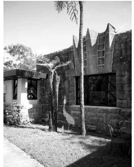
The southern facade features stone voussoirs as on the eastern facade, whilst the kitchen mirrors the verandah on the north-eastern side of the house. Photo: Chris Elfes
