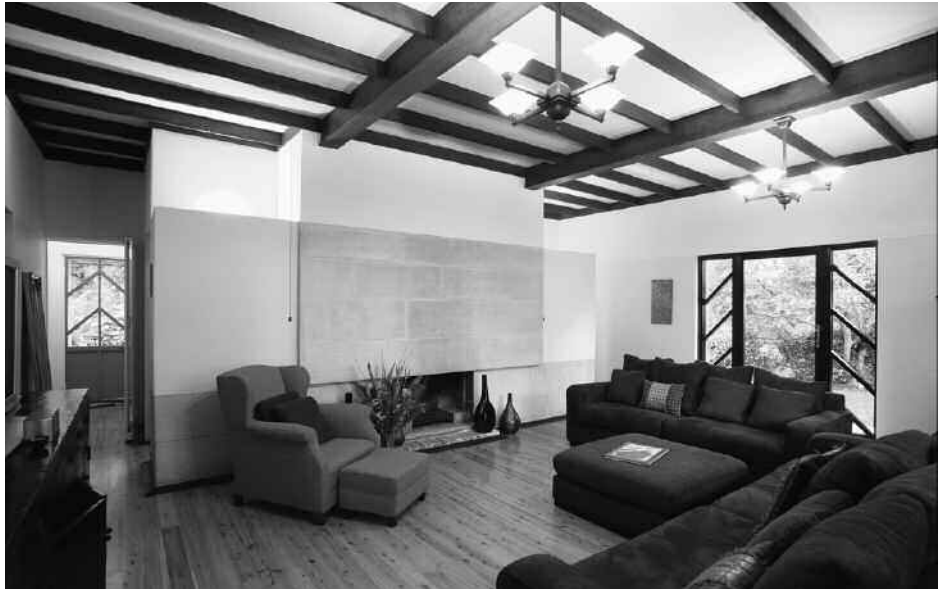
The living room with the restored sandstone fireplace. The 1970's aluminium sliding doors were replaced with a pivot door to match other window detail of the house. The exposed timber ceiling beams were also replaced to original detail. Photo: Chris Elfes
